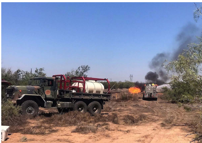
Figure 5. First pipeline rupture after 45 min. of blowdown, Midland County, Texas, USA.
