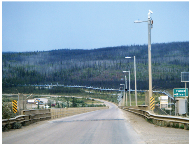
Figure 3. Author's photo of Trans Alaska pipeline at Yukon River crossing, July 2012.
